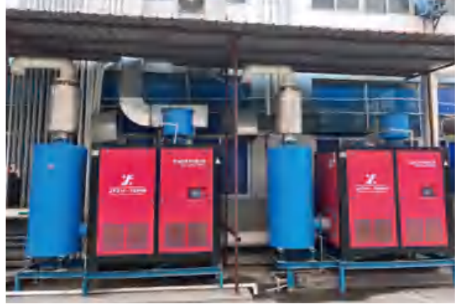
New Ventilation Facilities
