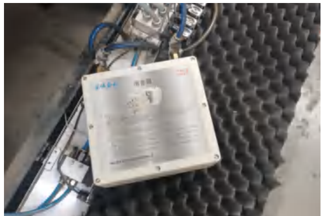
Silencers were installed to vacuum sound-emitting components
